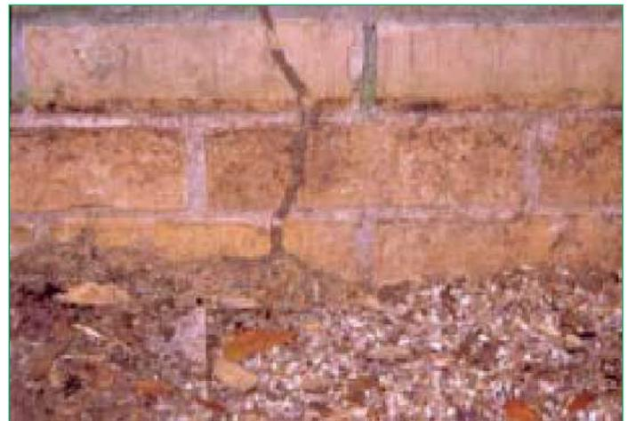
Figure 6. Subterranean termite shelter tubes on foundation wall.
